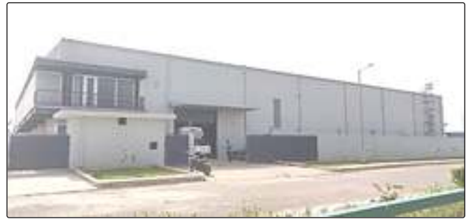
M/s Mercury Heatex Pvt. Ltd. (Factory Operational...)
