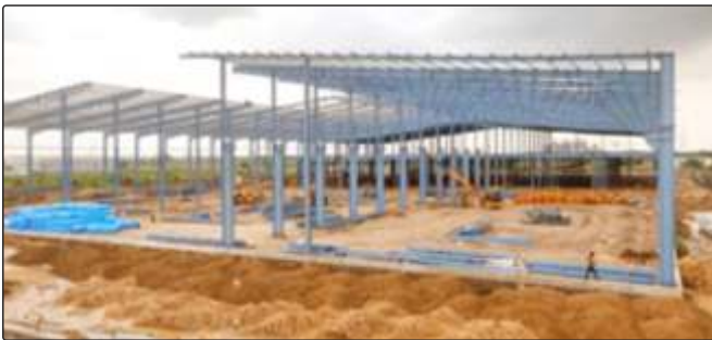
M/s EPACK Durables Solutions Pvt. Ltd. Factory under construction
