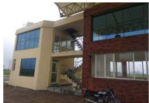
Main Gate House & Security Booth ...
