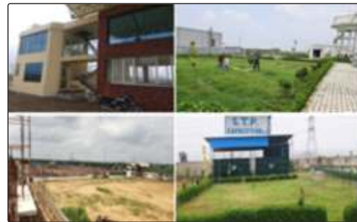
Gate House, Water Storage Tank, Fire Pump House & STP Area...
